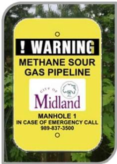
Pipeline markers like these are used to indicate the approximate location of the landfill gas pipeline and to provide contact information. Markers should never be removed or relocated by anyone other than a pipeline operator.
